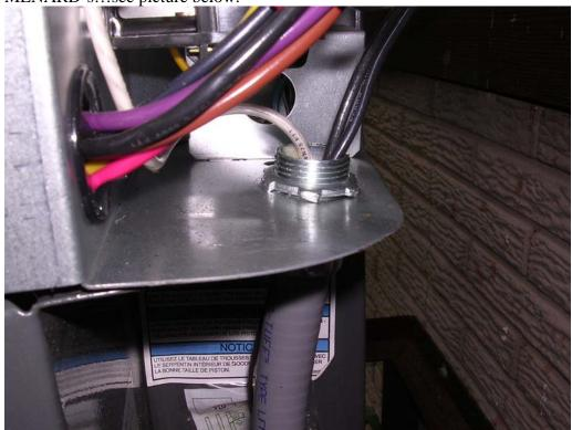
4. Make sure ALL your connections are TIGHT!....the BLACK wires connect to the 2 available screws...make you sure you are using the correct gauge wire....I am using 10 for example... you also need to connect to the thermostat...you can use wire nuts for that
