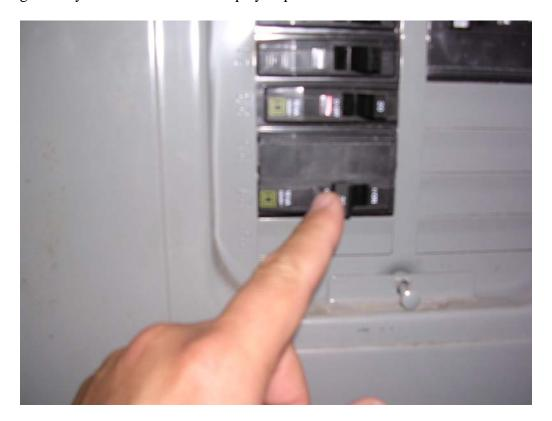
2. You will have to work outside as well as inside on this job so I choose to do the out side part first....I had an electrician install a 220V SEPARATE circuit and outside box in advance...notice have you essentially have 2 110V lines...see picture below...
